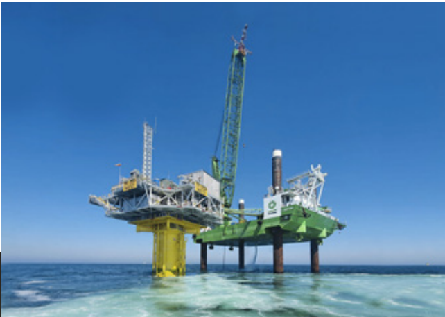
The Triton Knoll wind farm has been under construction off the North Sea coast of England since 2020. Scheduled for completion in 2022, it has already begun to supply electricity. The facility includes two transformer platforms (right) as well as 90 wind turbines mounted on the sea floor using monopiles (below).
