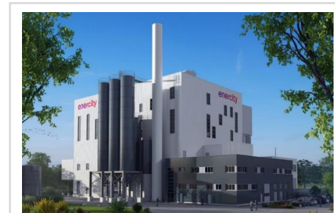
Helaba financed sewage recycling plant with green loan
